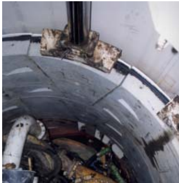
View into the tunnel and to one of the propulsion presses
