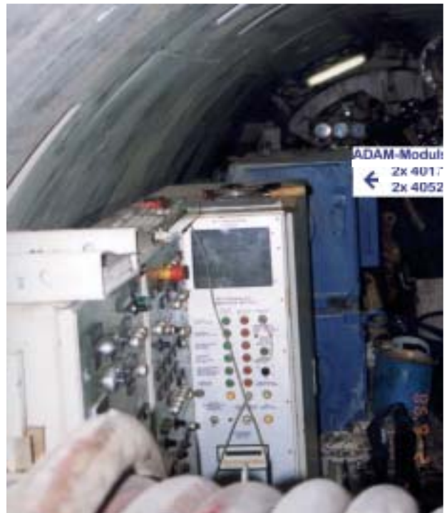
The control post
